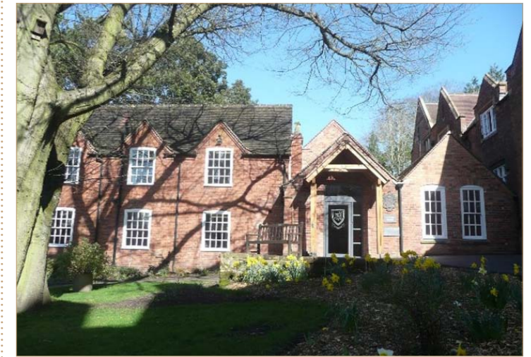
Lupton exterior after the 2016 refurbishment - photo by AGM, March 2017
