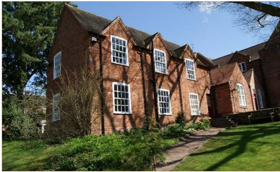
Lupton's base on campus 2010, previously School House Cottage, including the '93 extension on the right
